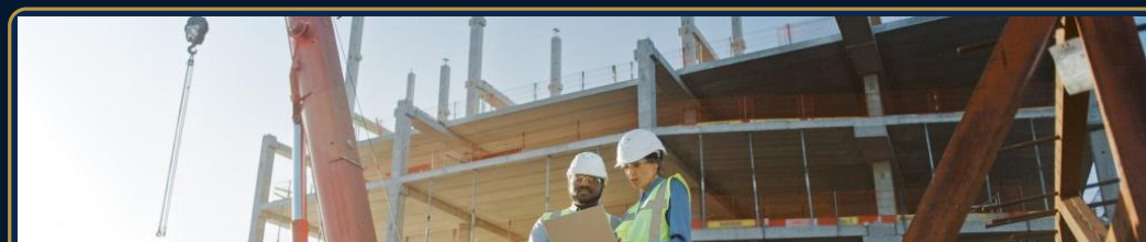
Site Execution / Delivery
