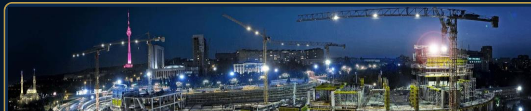
Civil Works / Construction
